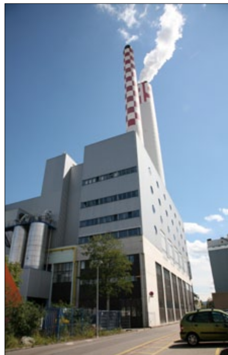
KVA waste-burning plant (Photo: IWB)
